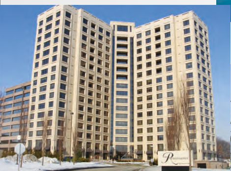
Apartments & Commercial Buildings
